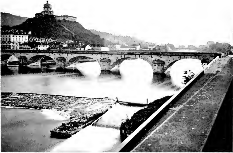
BRIDGE OVER THE PO, TURIN, ITALY.
